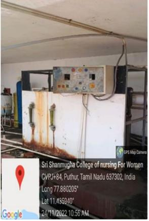
Water produced by reverse osmosis may be used for a variety of purposes, including desalination, waste water treatment, concentration of contaminants, and the reclamation of dissolved minerals. It is a water purification process that removes ions, unwanted molecules and larger particles from drinking water using a partially permeable membrane.
